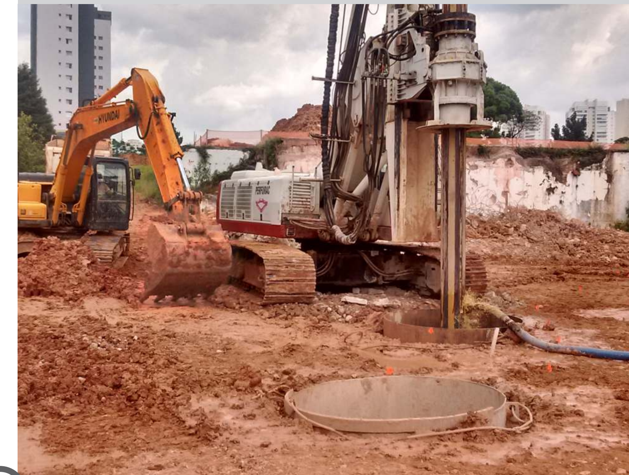
8ft diameter x 100ft depth boreholes
