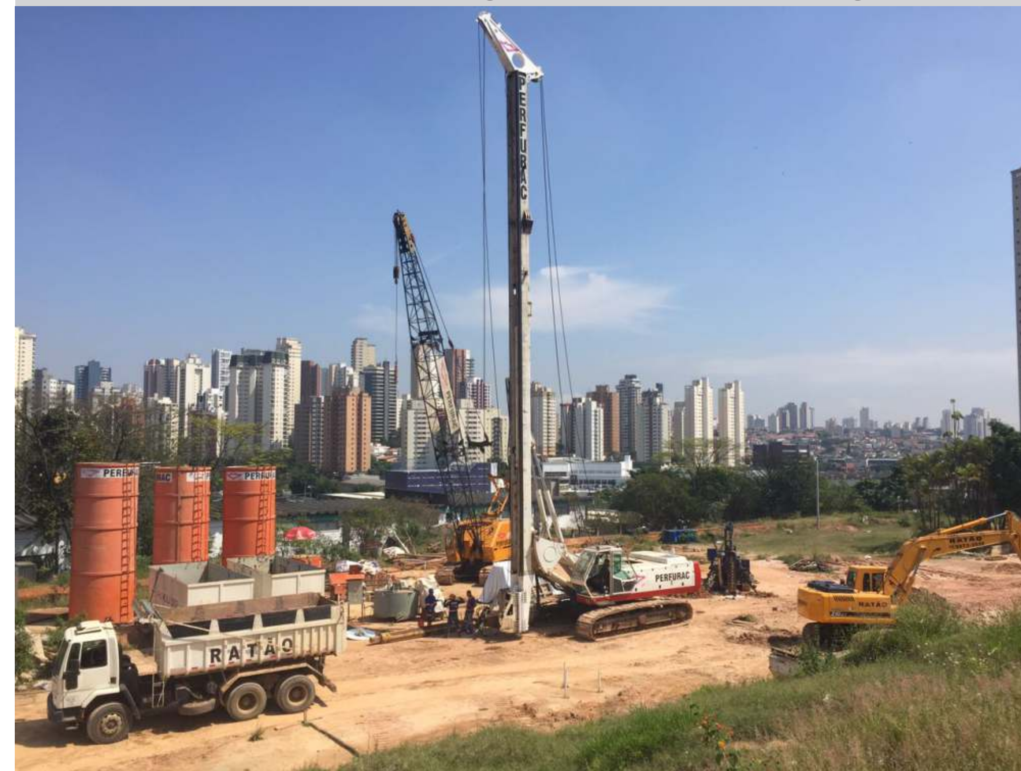
Modified large foundation rig
