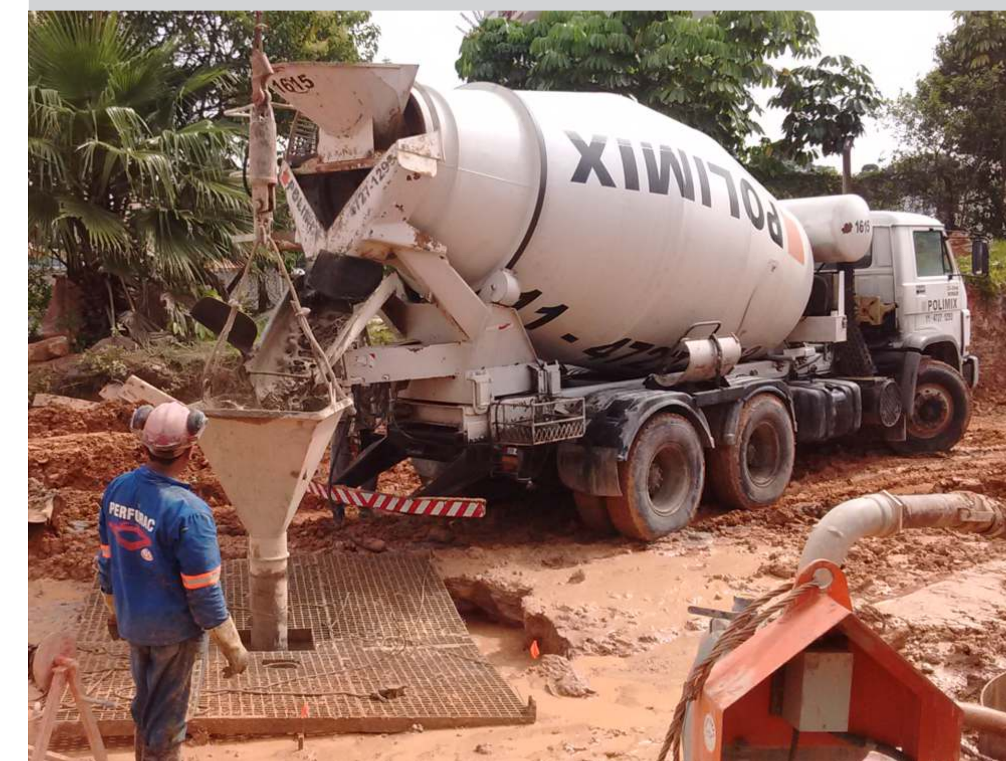
Cement filled boreholes
