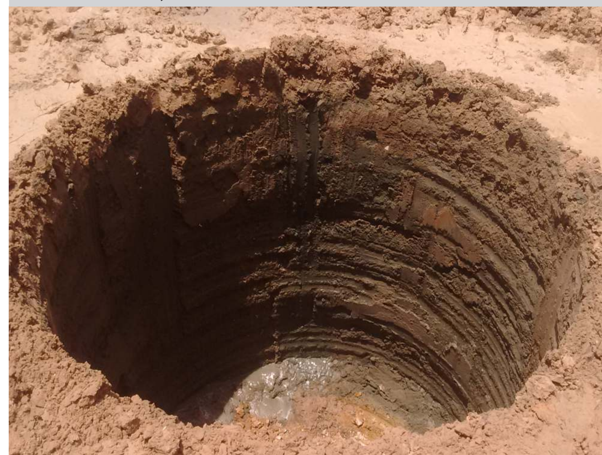
24,300 ton of soil removed
